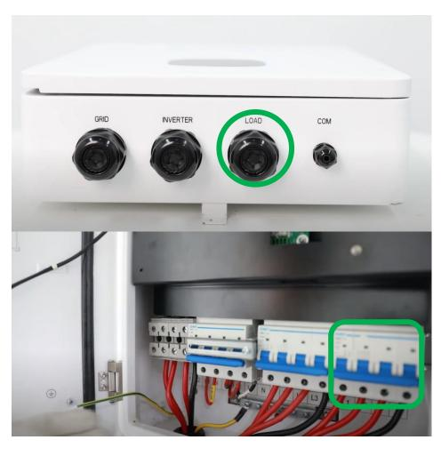
The third cable grommet is used for the backup circuit, see figure. The wires L1, L2, L3, N are connected to the circuit breaker called LOAD. A cable lug is to be pressed to the PE wire and connected as shown on the figure.
