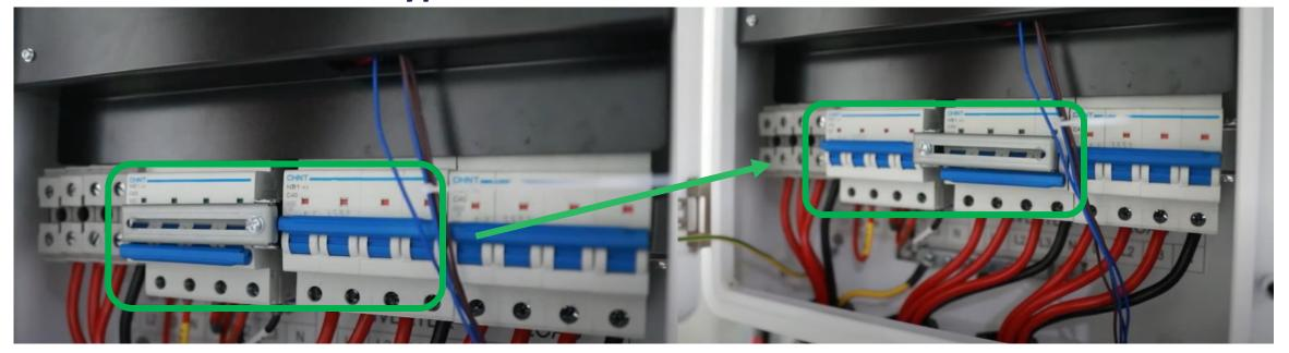
In case of SYN device failure, manual switching to BYPASS is required
