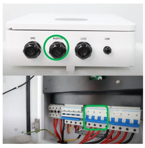
For cable connection of the inverter and the SYN device a second cable gland is used, see figure, and connect the wires L1, L2, L3, N to the circuit breaker called INVERTER. A cable lug should be pressed to the PE wire and connected as shown on the figure.
